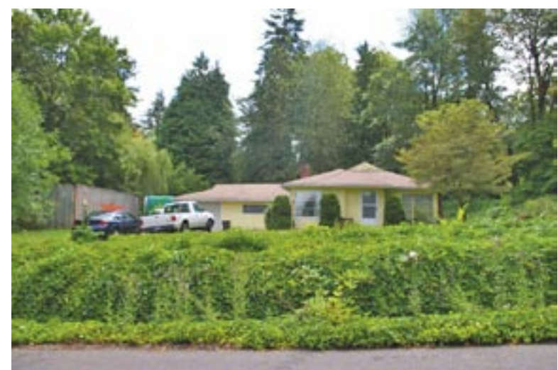
"Whitaker Heights." This lot will be divided into 5 lots with a street and sidewalk. 2 of the lots are only 6,000 sq. ft. This is in an R10 residential area of 50's ranch homes. The preliminary plans for the home show huge multi-story houses with dormers.
