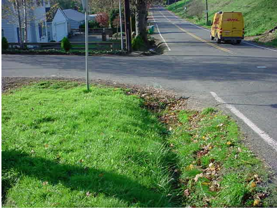
Figure 17. Existing Ditch, SE Corner of 45 th and Hamilton
